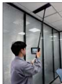
ceiling duct inspection
